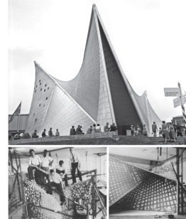
Philips Pavilion, Le Corbusier, 1958 The pavilion was composed of 9 pre-stressed concrete hyperbolic paraboloids, poured offsite.
